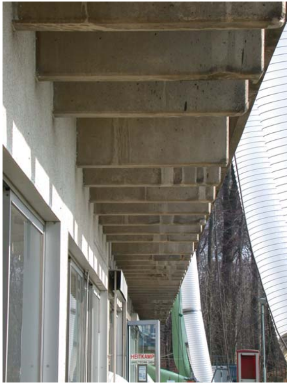
Figure 5 : Thermal bridges caused by brackets under the escape balconies.
