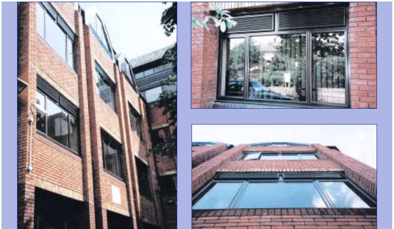
Figure 1: Air is drawn into the building by motorised Passivent window inlets sited within window frames.
