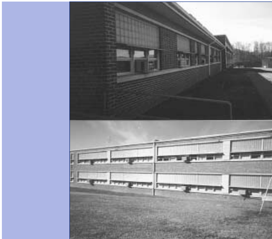
Figure 1: Akard elementary school. Top: North side Below: South side
